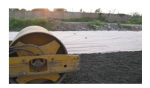
Compaction of gravel on secugrid 40/40
